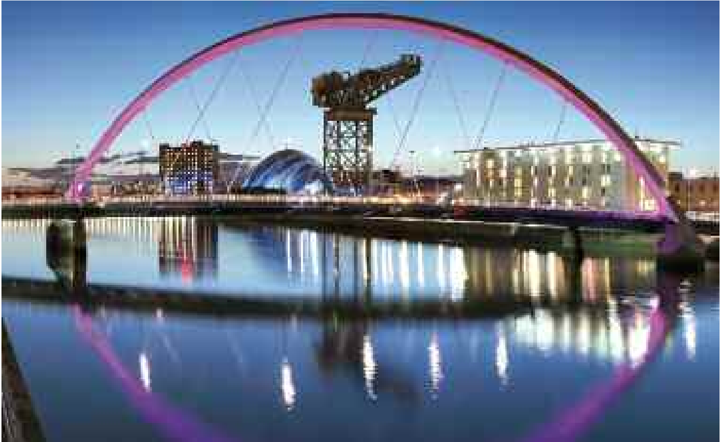
MODERN CITY: Glasgow's 'squinty bridge', aka the Clyde Arc Bridge, with the Scottish Exhibition and Conference Centre behind (centre)
